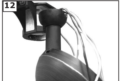
Hang assembled fan from the mounting bracket installed to ceiling in previous step. Make sure the fan is hanging straight. Rotate fan until the tab on the Mounting bracket engages the slot on the Downrod Ball. This must be done to prevent the fan body from rotating when the blades are in motion.
