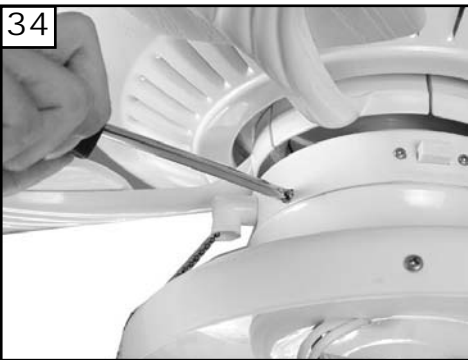
34 Attach switch cap to fan by lining up 3 screw holes and installing the 3 screws removed and saved from earlier step. Tighten screws securely.
