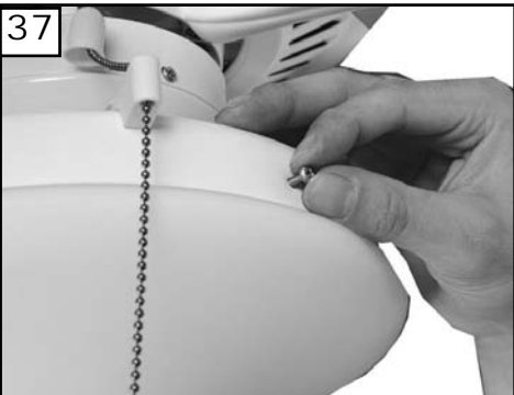
37 Push glass up into fitter and hand tighten the 3 screws to hold in place.
