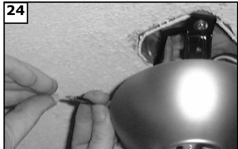
24 Make wire connections to power source using wire nuts provided. Make sure that no filaments are outside of the wirenut. After making the wire connections, the wires should be spread apart with the grounded conductor and the equipment-grounding conductor on one side of the outlet box and ungrounded conductor on the other side of the outlet box.
