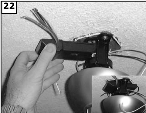
22 Install remote receiver by sliding into opening in the Mounting bracket. Make sure that the dip switches on the Transmitter and the Receiver are set to the same position. See Fig 39 for remote operation
