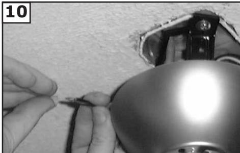
Make wire connections to power source using wire nuts provided. Make sure that no filaments are outside of the wirenut. After making the wire connections, the wires should be spread apart with the grounded conductor and the equipment-grounding conductor on one side of the outlet box and ungrounded conductor on the other side of the outlet box.
