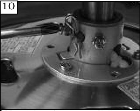
10 Tighten 2 downrod set screws and lock nuts.
