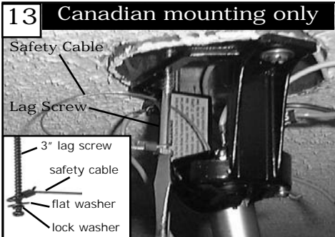
13 Canadian mounting only For Canadian installation in both flush and downrod mode the safety cable must be installed into the house structure beams using the 3" lag screws provided. Make sure that when the safety cable is fully extended the leadwires are longer than the cable and no stress is placed on the leadwires.
