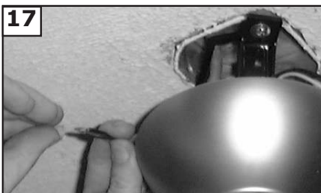
17 Make wire connections to power source using wire nuts provided. Make sure that no filaments are outside of the wirenut. After making the wire connections, the wires should be spread apart with the grounded conductor and the equipment-grounding conductor on one side of the outlet box and ungrounded conductor on the other side of the outlet box.
