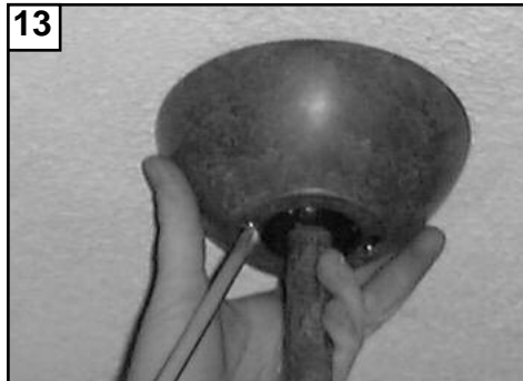
13 Raise the canopy up and align the two holes in the canopy with the two holes in the hanger bracket. Secure with two screws provided.
