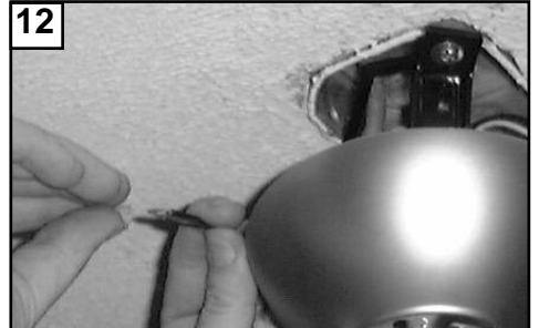
12 Make wire connections to power source using wire nuts provided. Make sure that no filaments are outside of the wirenut. After making the wire connections, the wires should be spread apart with the grounded conductor and the equipment-grounding conductor on one side of the outlet box and ungrounded conductor on the other side of the outlet box.
