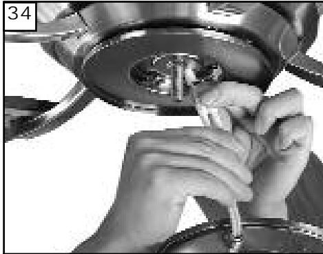
34 Plug white wire from fan to white wire from light kit. Then plug black wire from fan to black wire from light kit.
