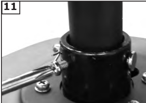
11 Tighten the 2 set screws on the yoke, once the down rod is in place.
