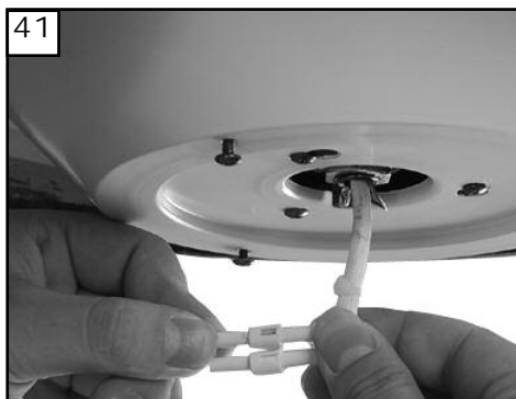
41 Plug white wire from fan to white wire from light kit. Then plug black wire from fan to black wire from light kit.
