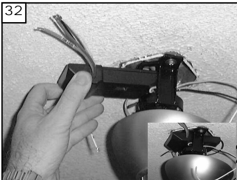
32 Install remote receiver by sliding into opening in the Mounting bracket. Make sure that the dip switches on the Transmitter and the Receiver are set to the same position. See page 7 for remote operation.
