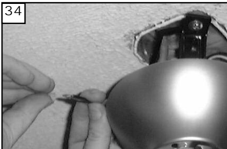
34 Make wire connections to power source using wire nuts provided. Make sure that no filaments are outside of the wirenut. After making the wire connections, the wires should be spread apart with the grounded conductor and the equipment-grounding conductor on one side of the outlet box and ungrounded conductor on the other side of the outlet box.
